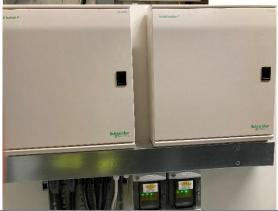
9. The existing earth wire to the SPDs in the comms room is undersized (greater than 6mm required). Rewire the earth in line with manufacturers instructions before handover as required by BS7671 2018. (Section 534).
