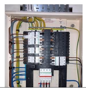
3. Surge Protection has not been fitted to existing reused DB's. Fit surge protection before handover as required by BS7671 2018. (Section 534) unless the circuits have no vulnerable equipment, or it has been excluded in writing.
